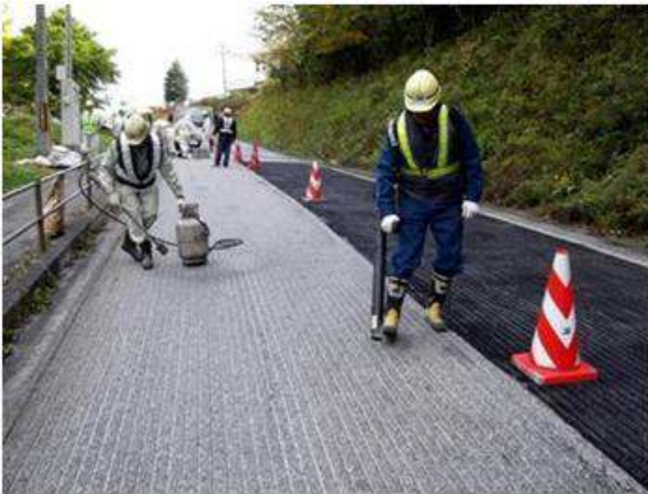
3. Cleaning the pavement
