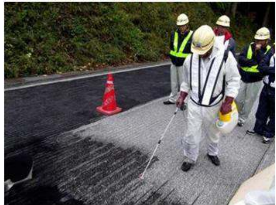
4. Applying a special adhesive agent
