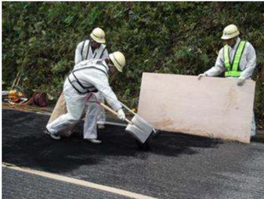
5. Spreading rubber powder
