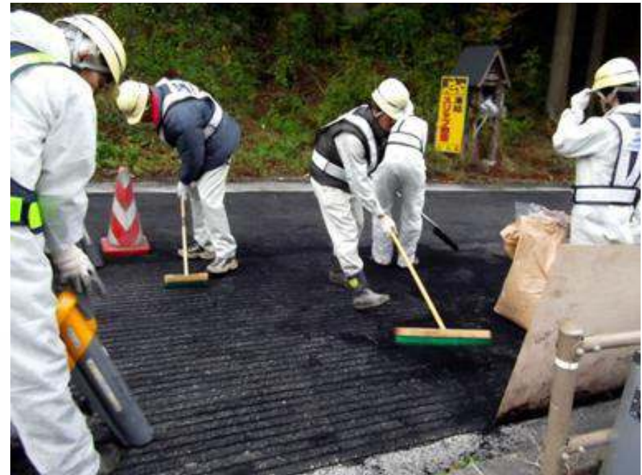
6. Removing and collecting excess rubber powder
