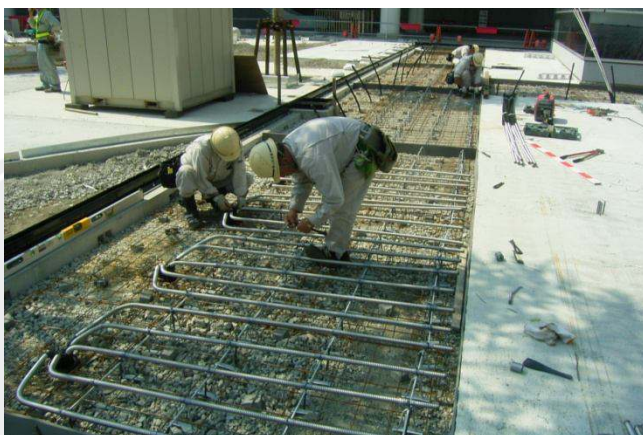
3) Heat pipe anchoring and paving
