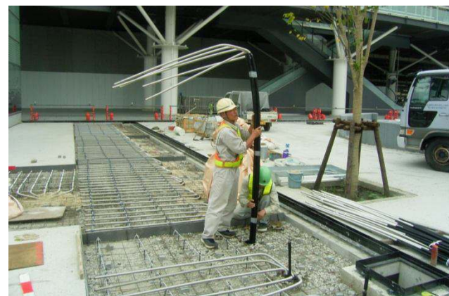
2) Heat pipe installation
