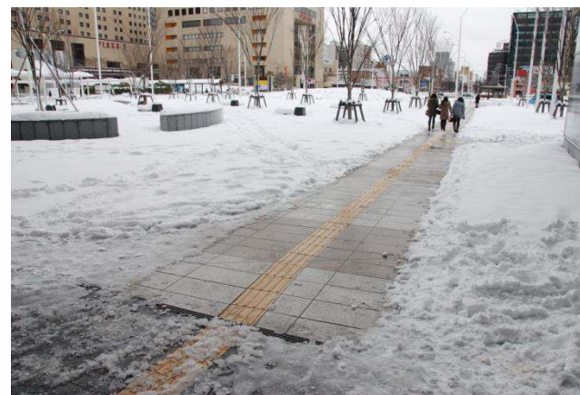
4) Completed for snow melting
