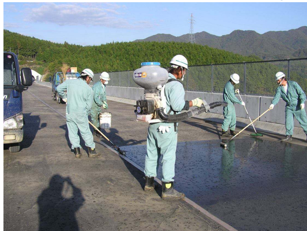
Top coating MMA: 0.2 kg/m 2 Non-skid Sand: 0.6 kg/m 2
