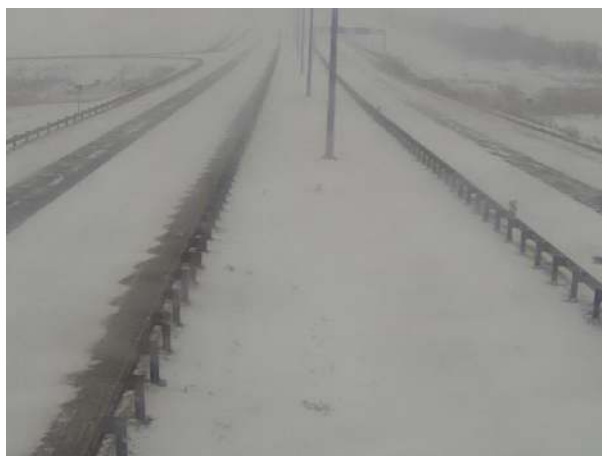
Figure 7 – Variants of crash barriers placement on experimental sites
