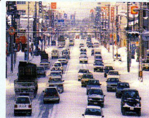
Post-installation (National Highway 12 in Asahikawa)
