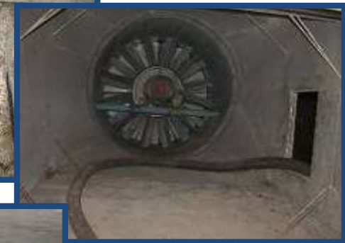
Mud Pumping in Ventilation plenums
