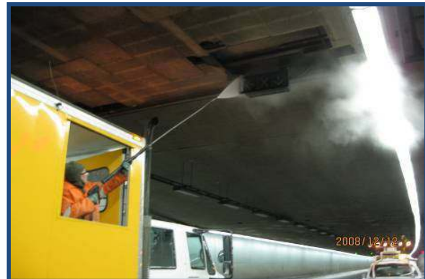
Winter Cleaning of lane Signals using a water jet
