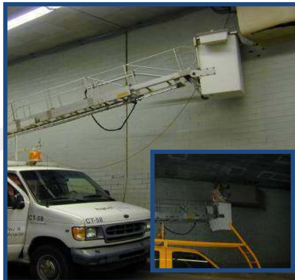
Camera in protective climate-controlled casing
