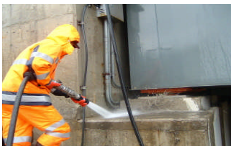
Figure 10 – High-pressure water cleaning
