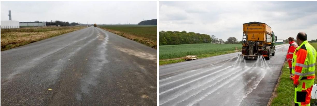
Figure 9 - Salt application (left: old pavement, right: new pavement)
