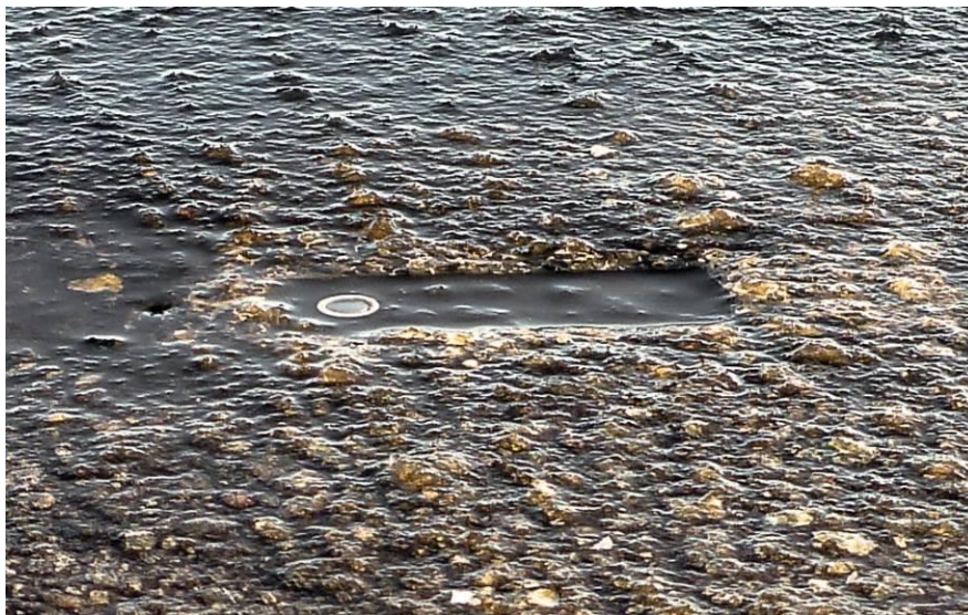
Figure 2 – Road surface condition sensor (Vaisala DRS511) installed in the pavement
