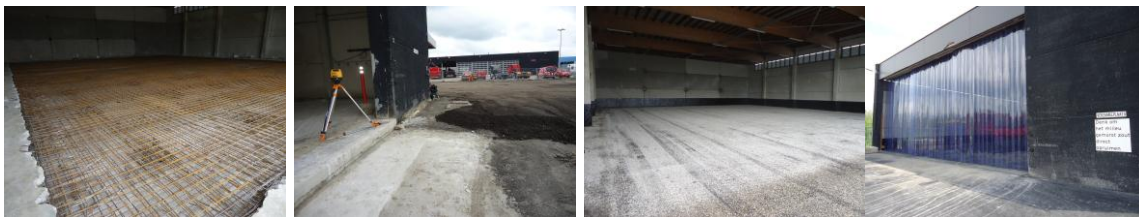
Figure 5 – Reconstruction of a salt storage building after decontamination. The floor is removed and replaced with leak-proof paving - the ground around the storage building is also restructured - a protective coating is applied to the walls inside the storage building - best practice procedures are adopted.
