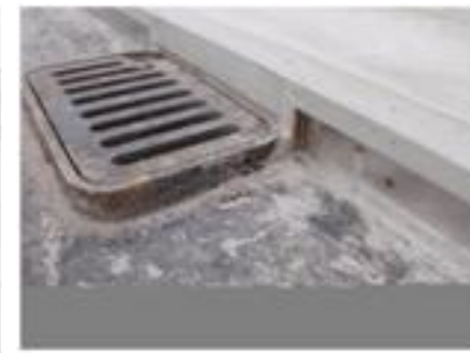
Picture 16-Connection to the bridge drain
