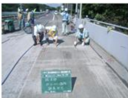
Picture 4- Sound inspection
