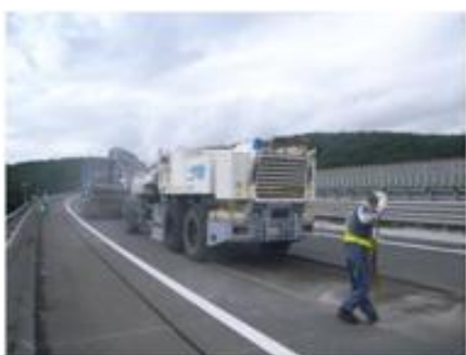
Picture 3- Cutting the road surface
