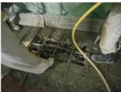
Picture 7-Base plate goes into sand state
