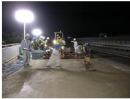
Picture 13-Pouring steel fiber concrete
