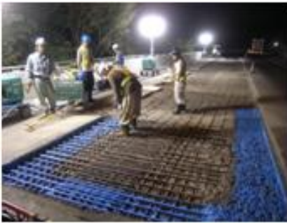
Picture 12-Applying joint glue
