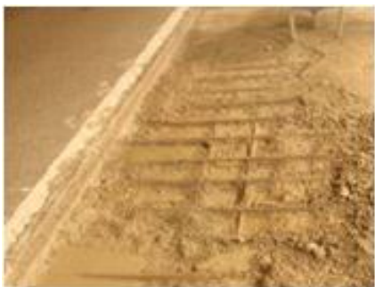
Picture 6-Stagnant water in the established base plate
