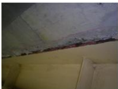
Picture2-Exfoliation on the primary plate
