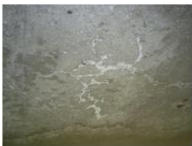
Picture 1-Free lime on the primary plate
