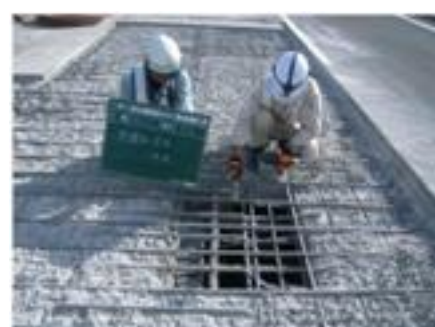
Picture 8- Defect of reinforcing bars
