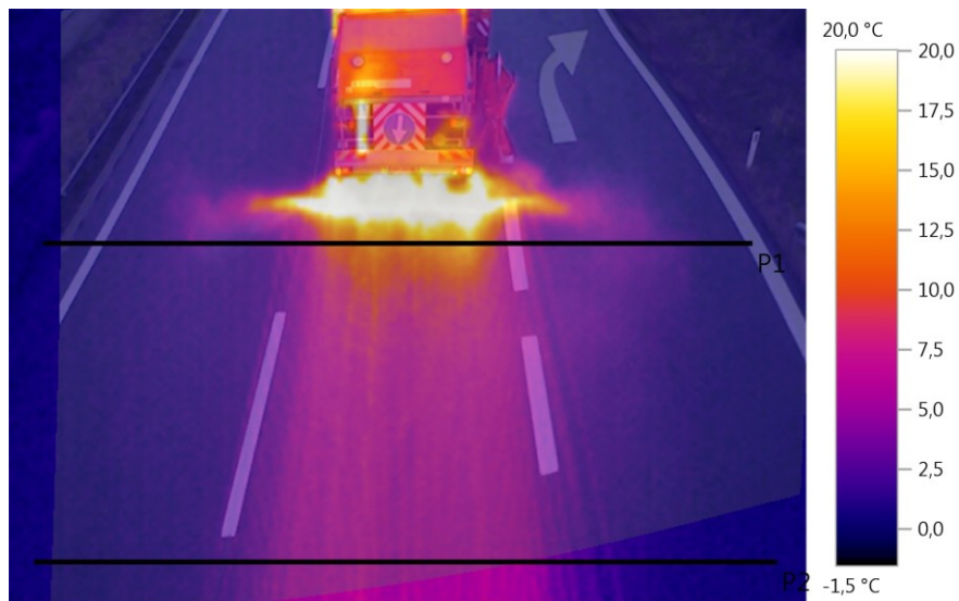
Figure 3 - Image of hot solution application taken with a thermographic camera.
