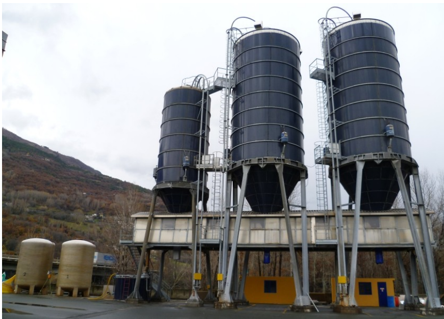
Figure 1 - Nus Maintenance Station
