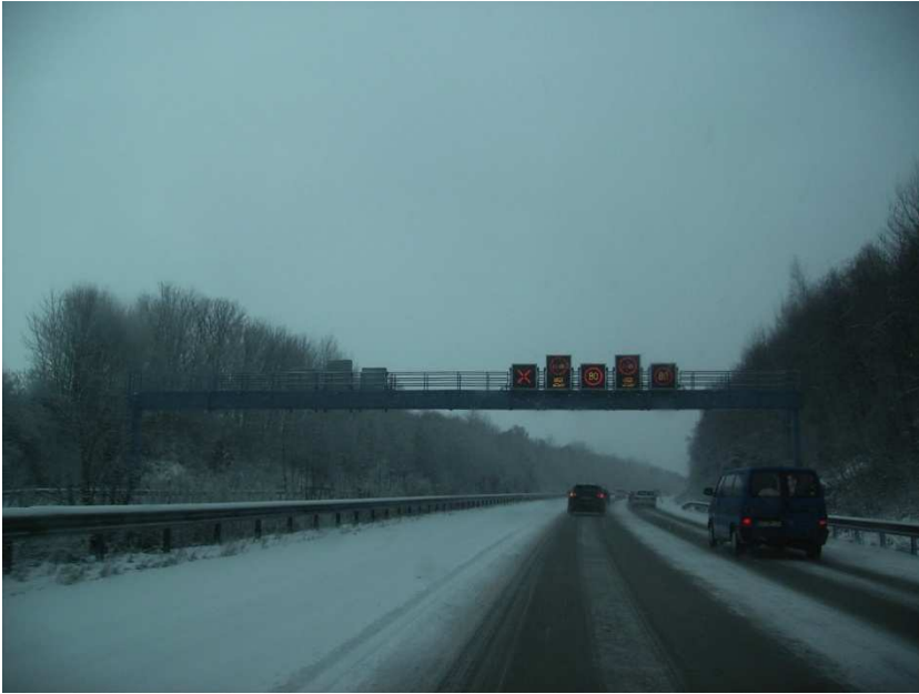
Picture 3: lane blocked by signs
