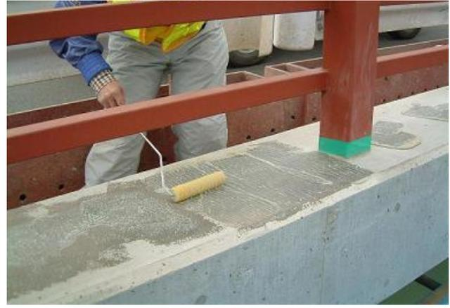
Photo 4 – A coating of silane surface penetrants is applied.
