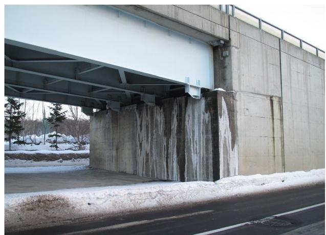
Photo 2 - Deicing salt supplied to a concrete structure
