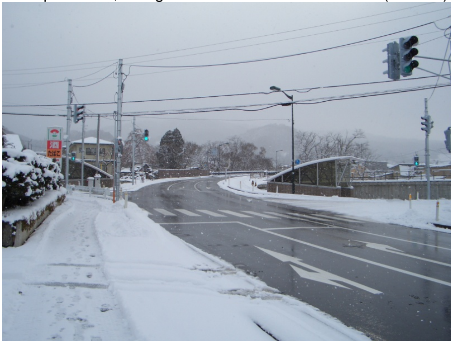
Photo 2 - Snow Melting System without groundwater sprinkling in Yamagata
