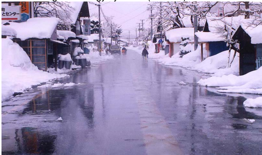
Photo 1 - Snow Melting System with groundwater sprinkling
