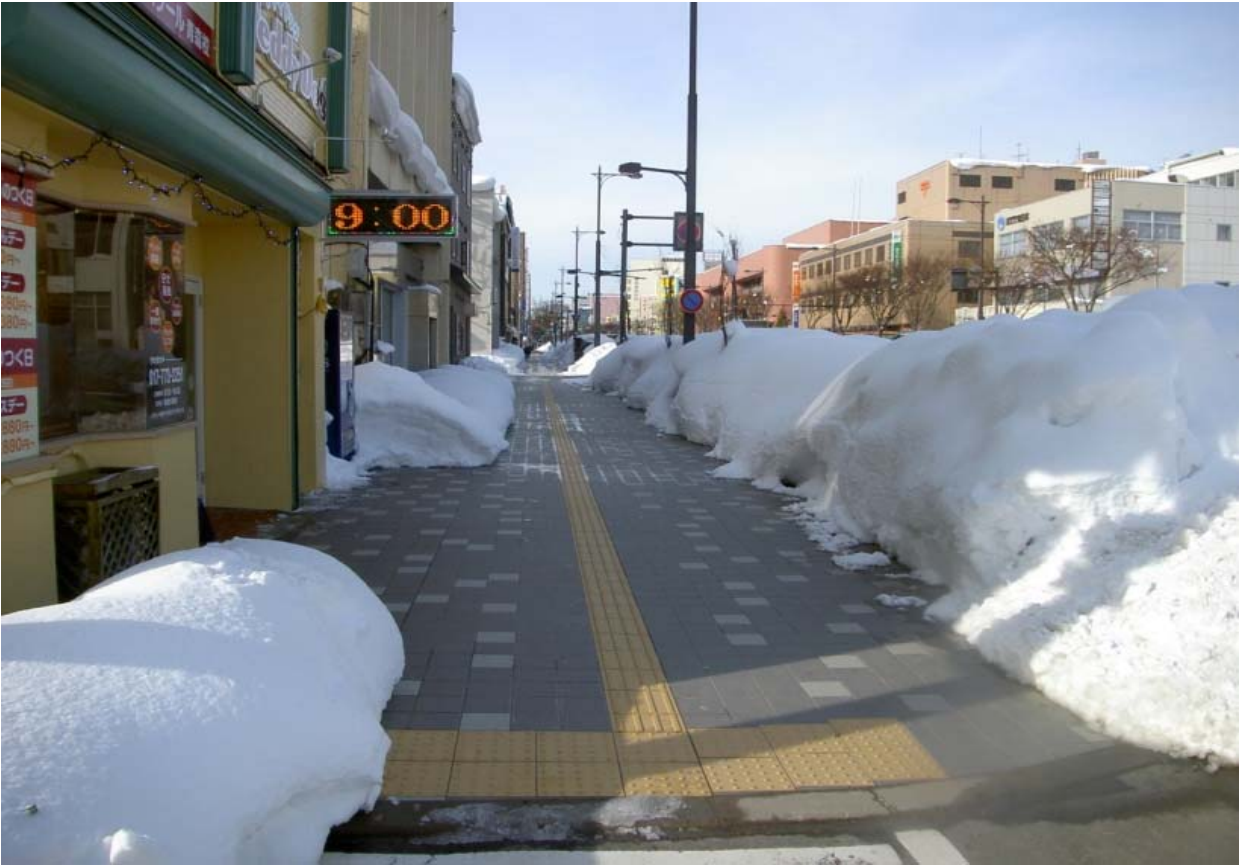
Photo 3 - SMS using ground source heat pump in Aomori-city
