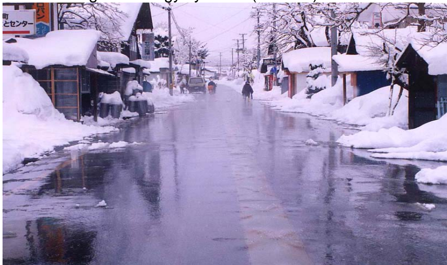
Photo 1 - Snow Melting System with groundwater sprinkling
