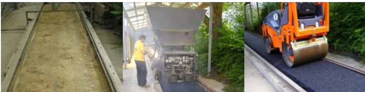
Figure 1 – Construction of asphalt mixture on the test track
