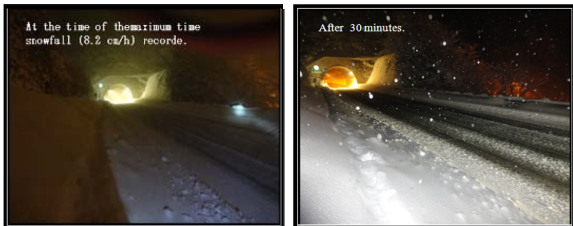
Figure 8 - Road condition of the Yakushi Tunnel
