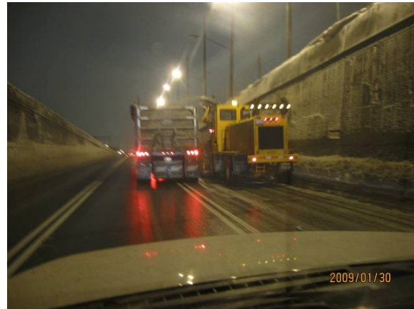
(b) Snow removal at the exit
