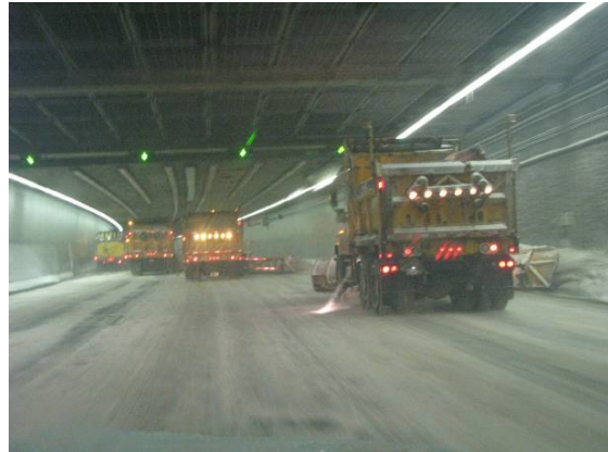
(b) Snow and ice removal inside a tunnel
