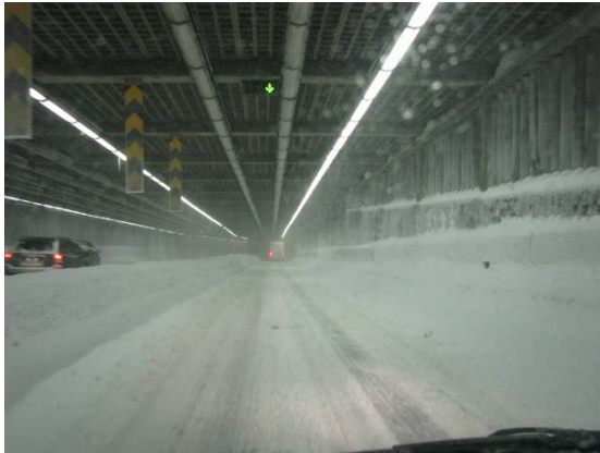
(a) Accumulation of snow at the portal
