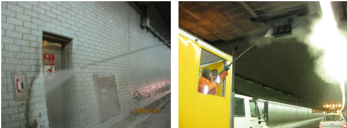
(a) Cleaning the signage
