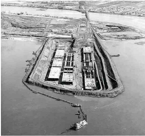
(a) Dry dock at the Lafontaine Tunnel
