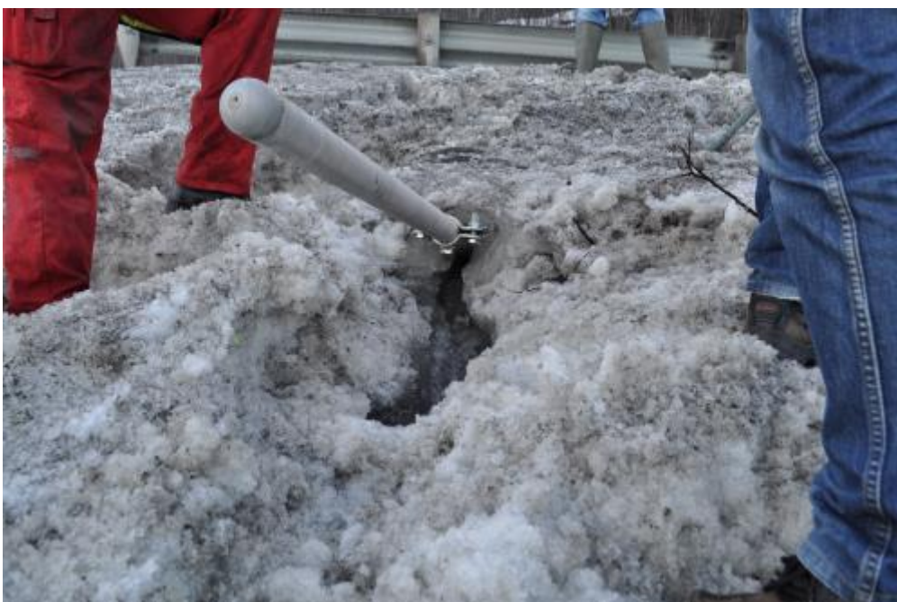
Picture 6 – Culvert outlet draining excess water Photo: Heatwork
