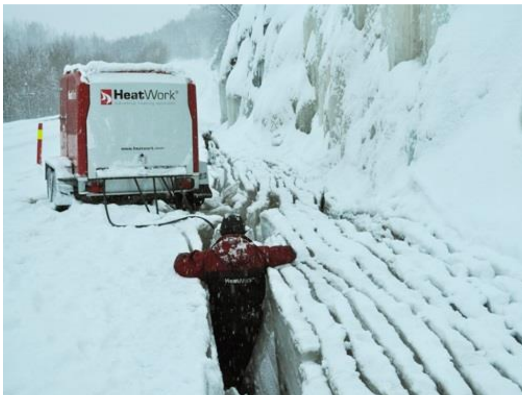
Picture 7 –Field testing heater hoses in frozen drain trench Photo: Heatwork
