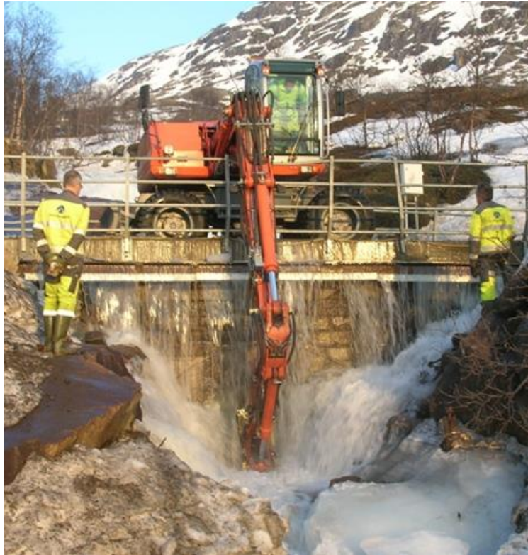
Picture 1 – Using excavator to remove ice from culvert outlet Photo: NNRA
