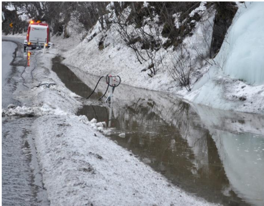
Picture 5 – Frozen culvert and drain trench with excess water
