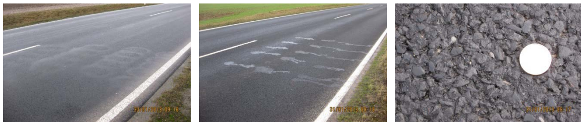
Figure 5 – Road B19 direction_A with wet (left) and dry (middle) surface conditions, close-up view of road surface (right)
