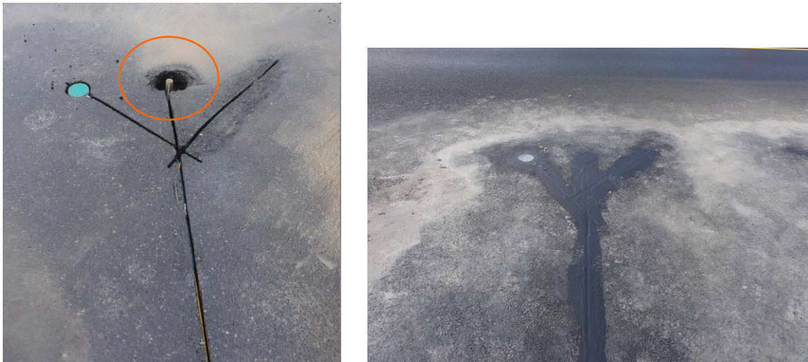
Figure 7 - Installation of the frost probe in the pavement
