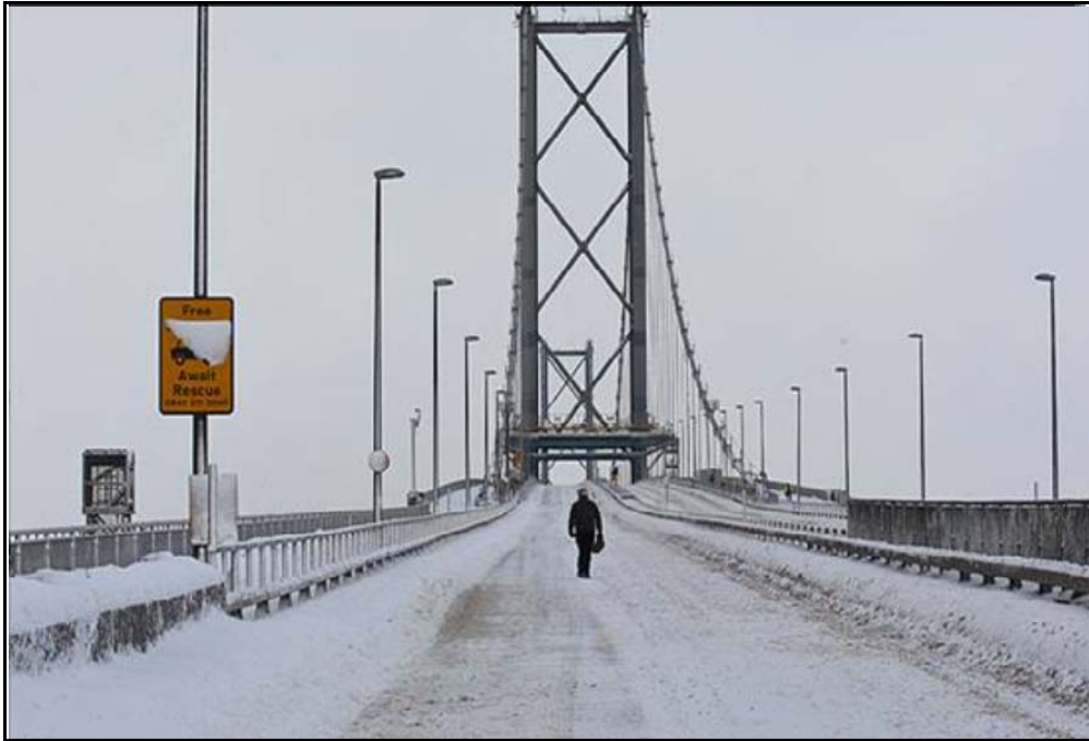
[Figure 4 – 2010/11 Conditions (Forth Road Bridge)]
