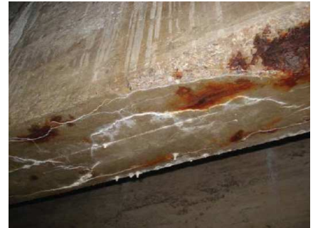
Figure 8. Structure nº 2; N-630, p.k 88
