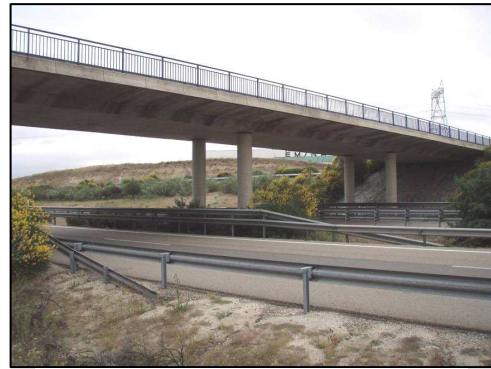
Figure 4 Bridges of type C
