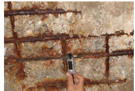
Figure 9. Structure nº 2; N-630, p.k 88
