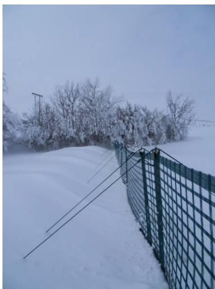
Photograph 4: Fageole Summit snow fence (Source: IRSTEA Institute)
