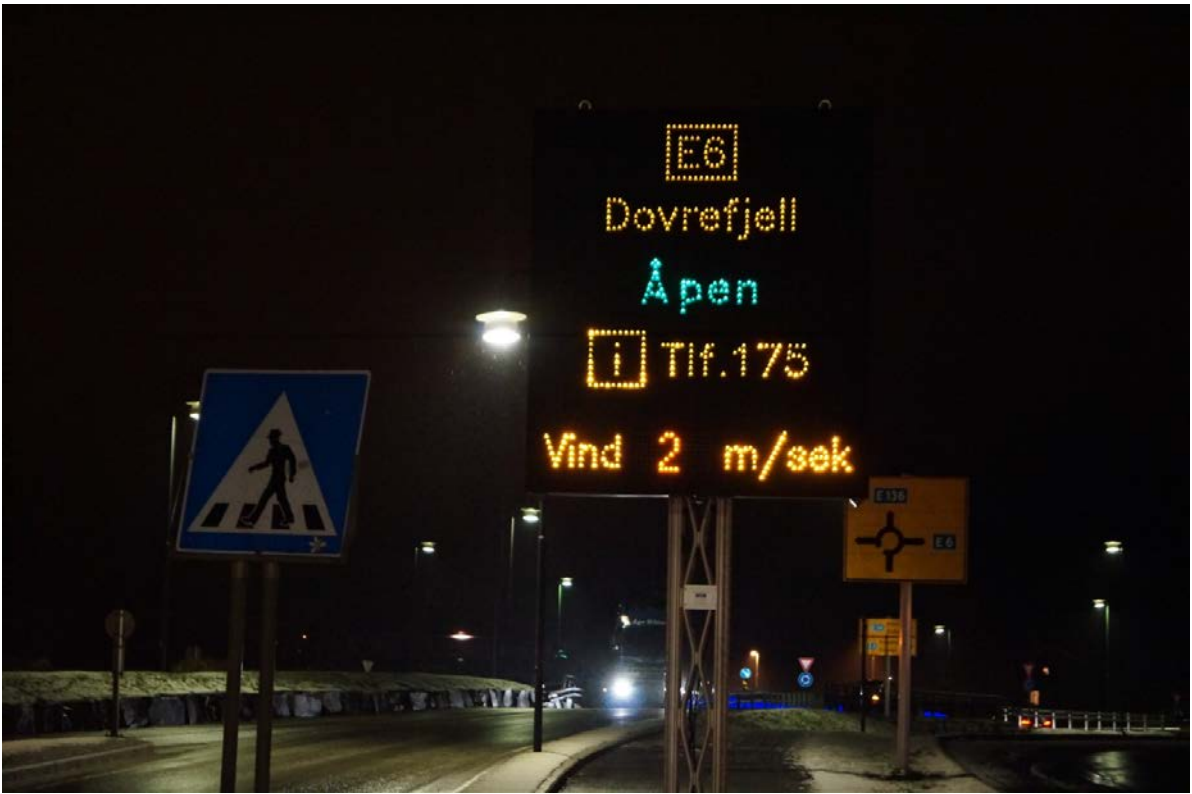
Figure 4 - Variable signpost in Dombaas. The sign says that the road is open and the wind strength is 2 m/sec.
