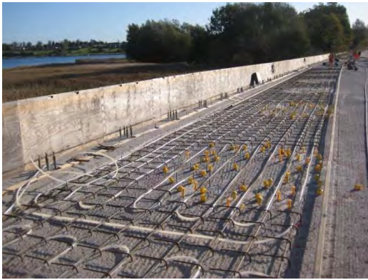
Fig. 16. Bridge deck with hoses for hot water.
