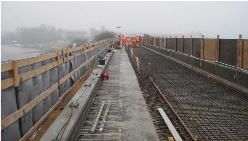
Fig. 8. Bridge deck with reinforcement for concrete overlayer
