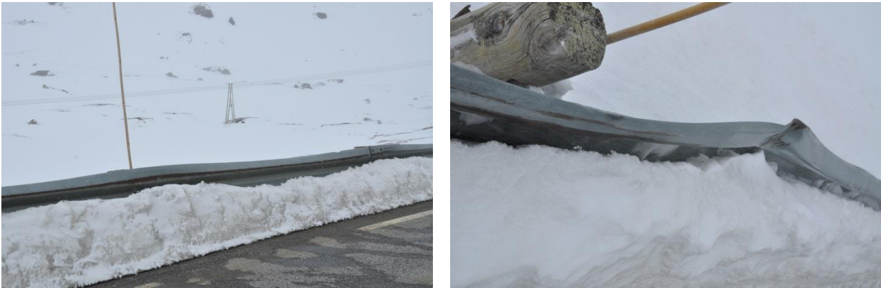
Figure 11: standard Norwegian safety barrier (wooden posts) on a mountain road in Norway
