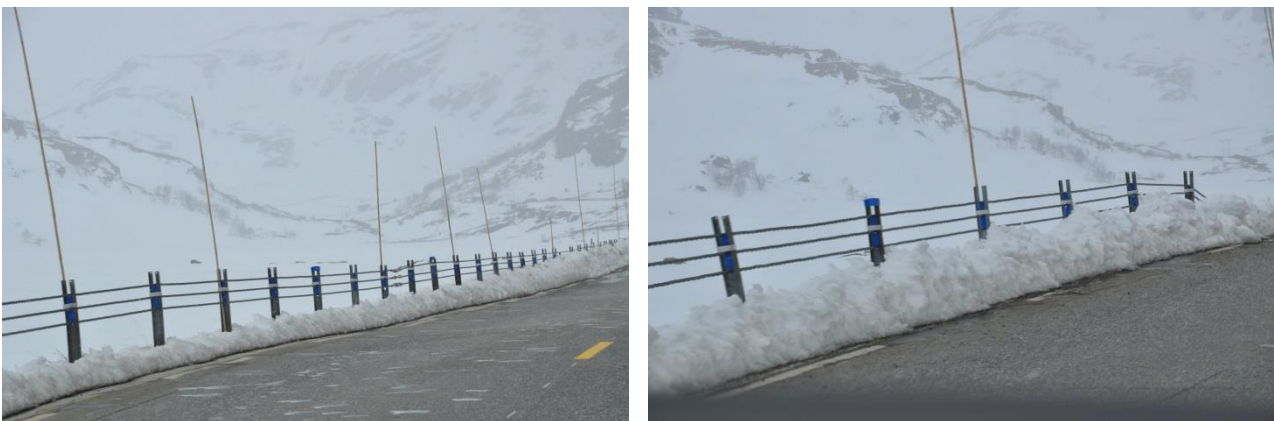
Figure 10: wire rope safety barrier on a mountain road in Norway
