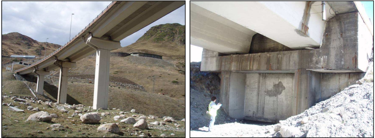
Figures n° 2 and n° 3. View of the viaduct to abutment n° 1 (left) and abutment n° 2 (right)
