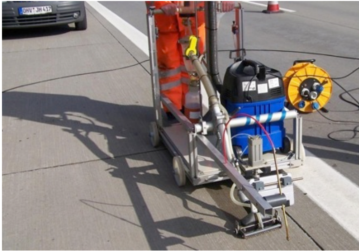
Figure 1: Collecting spreading material using the rinsing-suction device
