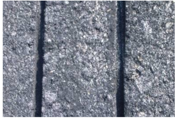
Photo 8 Surface of dense graded pavement after application of rubber powder (and grooving)
