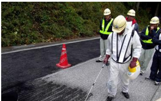
Photo 13 Application of the special adhesive agent
