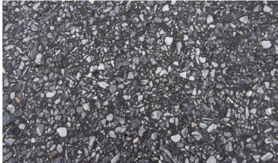
Photo 11 Existing pavement surface before rubber powder application
