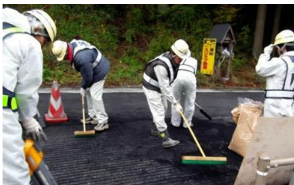
Photo 15 Removing excess rubber powder
