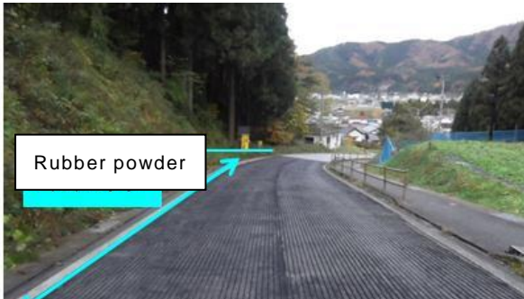
Photo 17 Rubber-powder freezing prevention pavement (dense graded asphalt + grooving)
