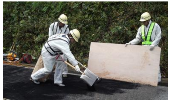
Photo 14 Spreading rubber powder
