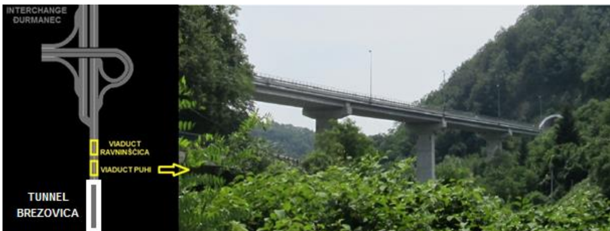
Photo 3 – Viaduct Puhi (227 m)
