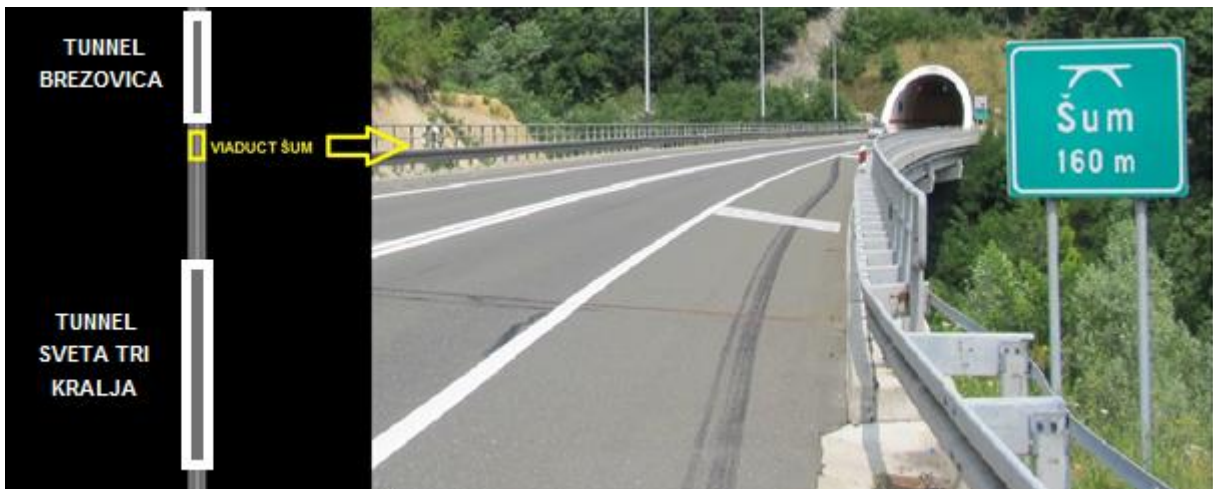
Photo 2 – Viaduct Šum (160 m)
