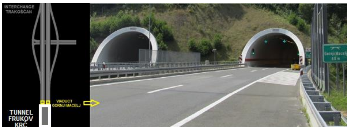
Photo 5 – Viaduct Gornji Macelj (60 m)
