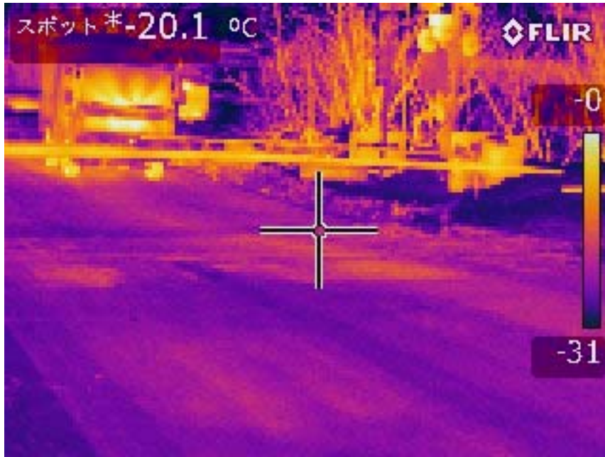
Figure 4 - Two sides of a railroad crossing
