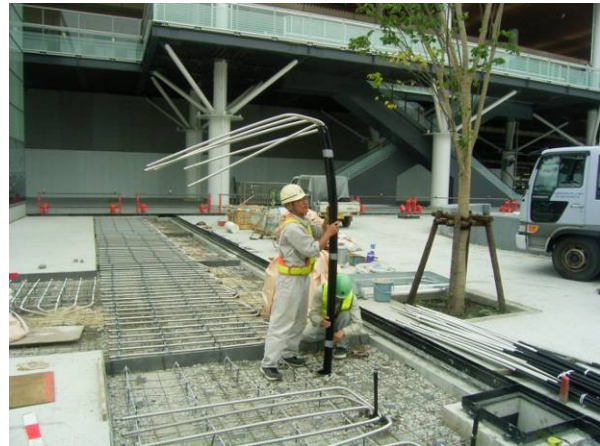
b: Heat pipe installation
