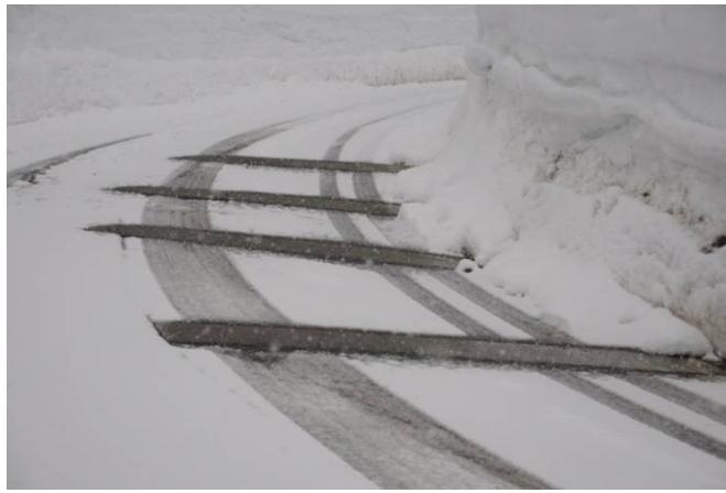
Figure 16 - Partial installation at a steep slope to prevent skidding accidents
