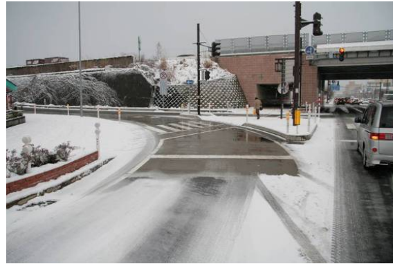
d: Carriageway (interchange ramp/curve)
