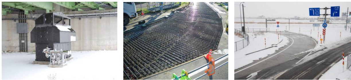
Air-source heat pump
