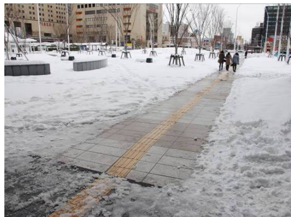
d: Completed for snow melting
