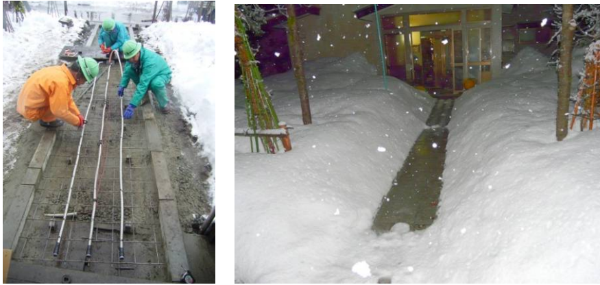
Figure 17 - DME heat pipes and snow melting
