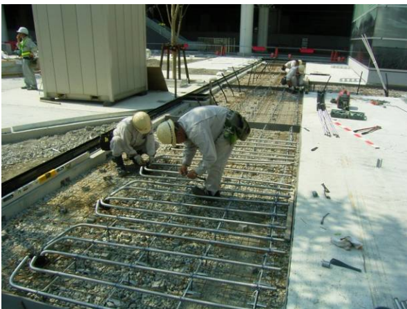
c: Heat pipe installation and fixation
