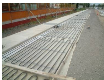
Radiation pipes
