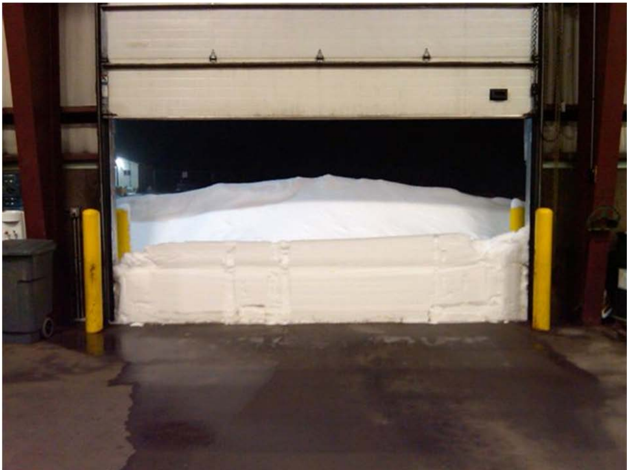
Figure 3: Drifting at Facility Access Point in McHenry County
