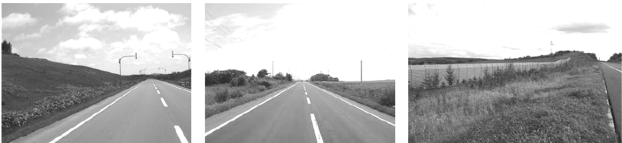
Figure 4 - Snow-control by road structure modification: drift-free cut (left); drift-control embankment (center); gently sloped embankment (right)
