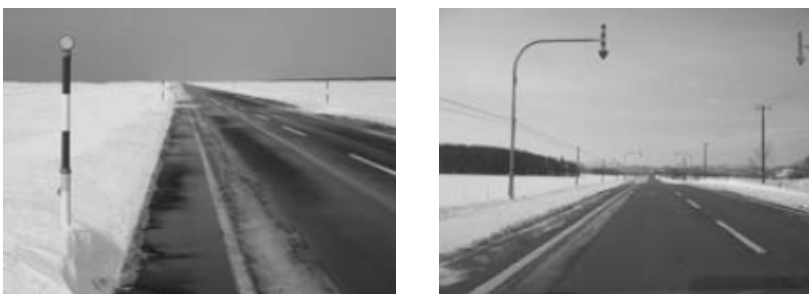
Figure 5 - Delineation facilities: snow-pole (left); fixed-post delineator (right)
