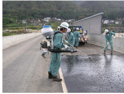
Spraying anti-skid sand
