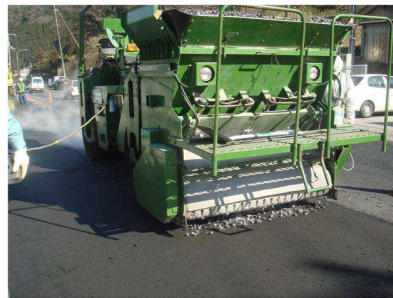
Chipping and breakdown rolling
