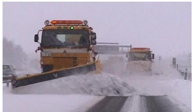
Photo 1: Snow Removal Work in Tohoku
