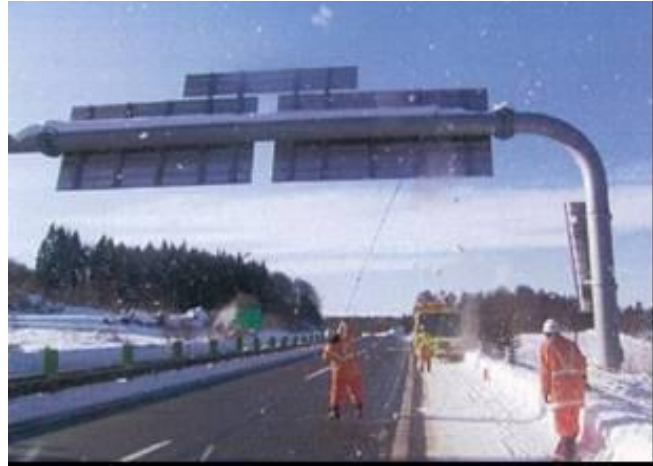
Photo 3: Snow Removal Work for Preventing Snow Drop
