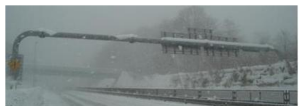
Photo 2: Snow Accumulated on Road-sign Post
