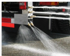
Fig. 3 - Spreading up to 5 lanes by spray bar and nozzles
