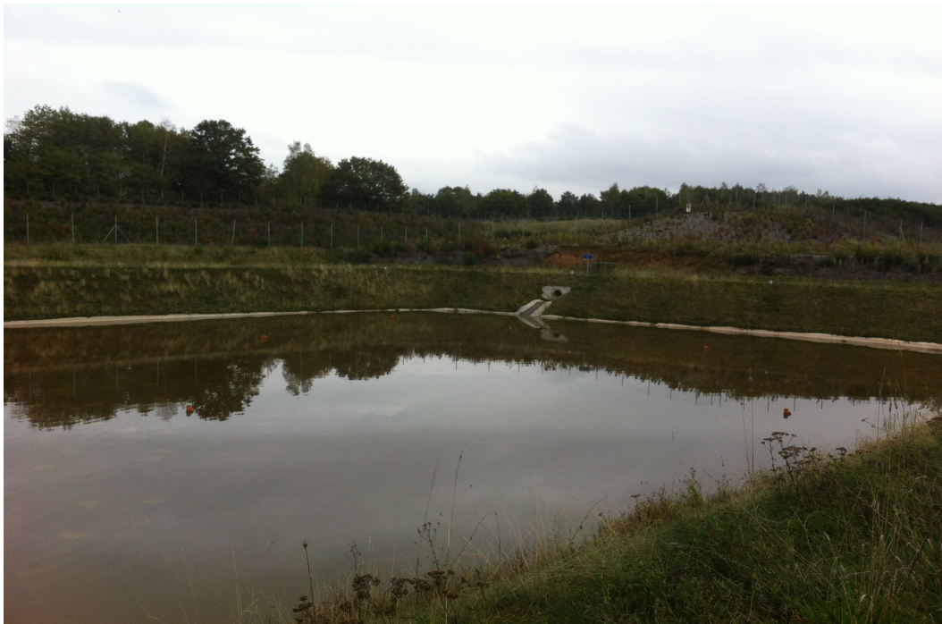
Figure 2 - Photography of Chenevières pond.
