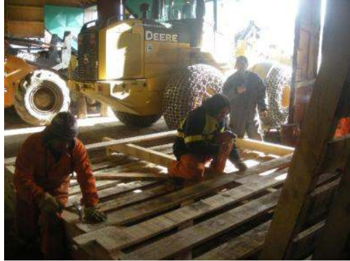
Figure 10 - Construction of panels
