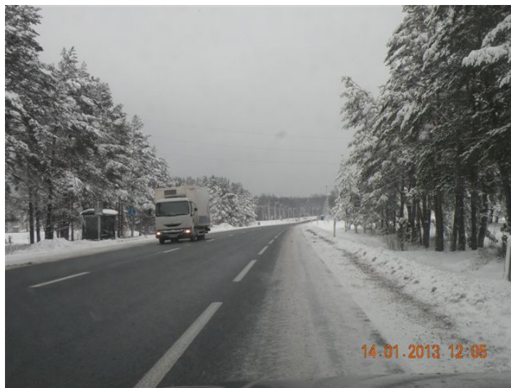
Figure 7 - Road with paved shoulders.
