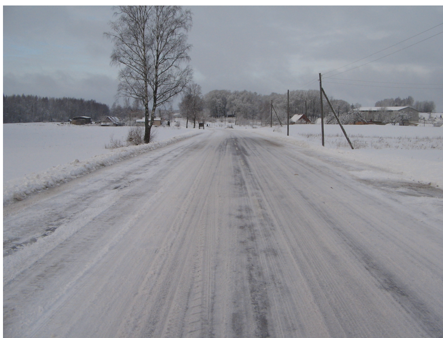
Figure 4 - Maintenance classes A and A1 in changing weather conditions
